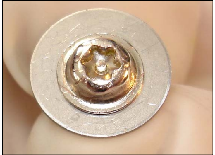
6. Security torx screw detail.
